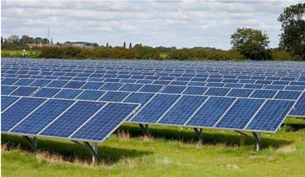
Figure 11: Single axis tracking solar farm with bi-facial panels 7
