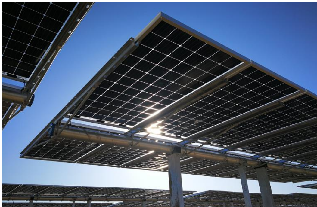
Figure 11: Single axis tracking solar farm with bi-facial panels 7
